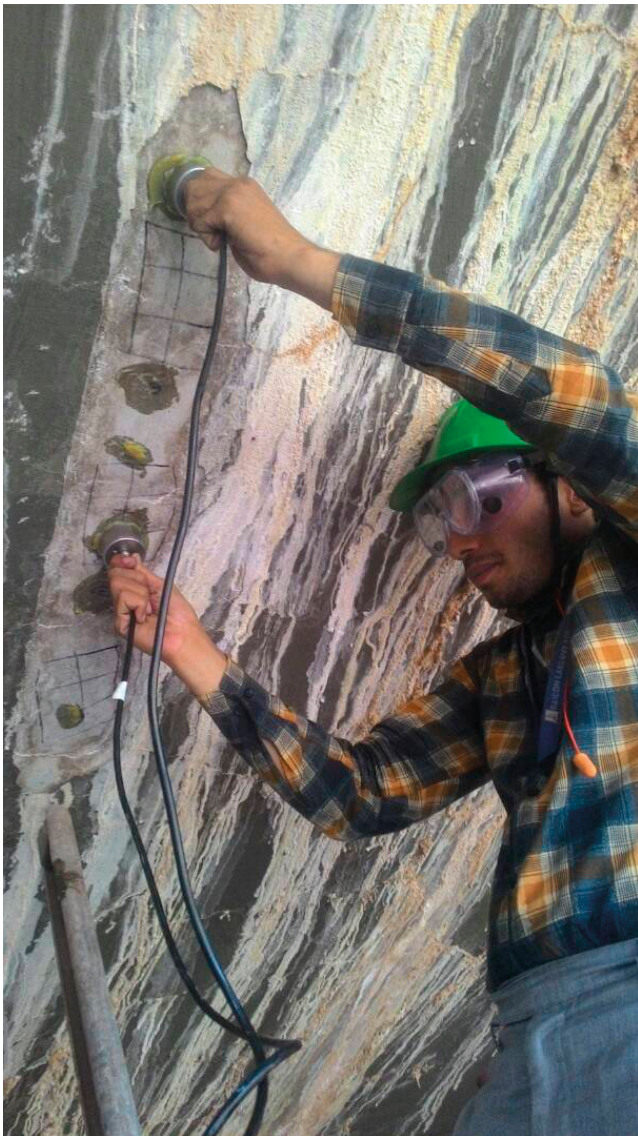
Figure 2. Ultrasonic pulse velocity test
