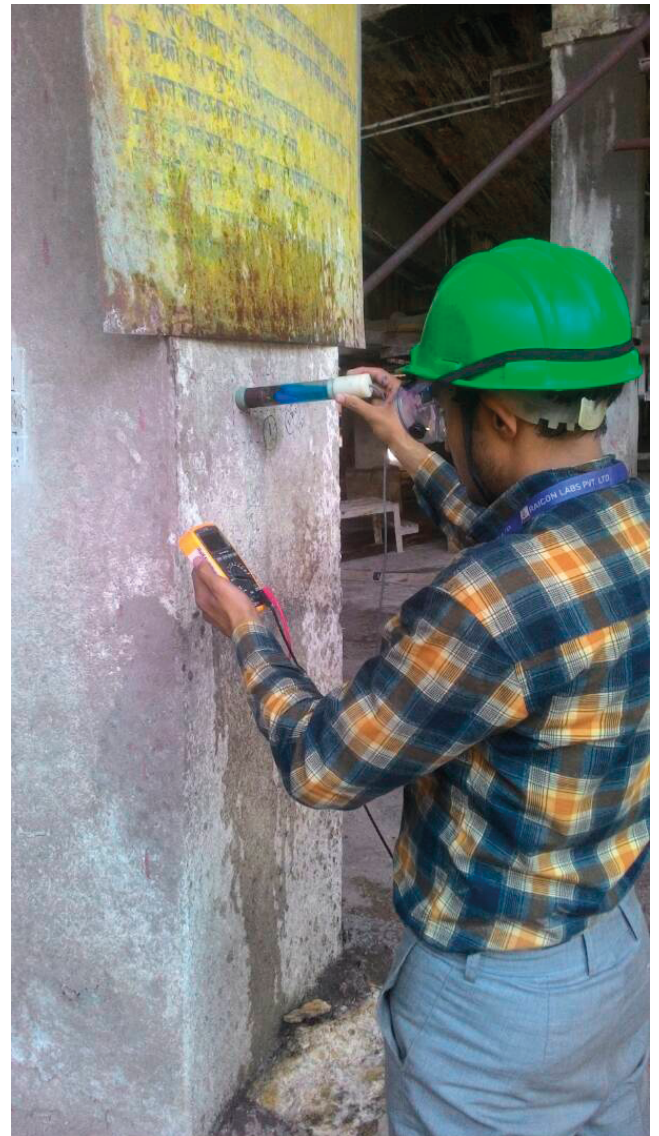
Figure 3. Half Cell Potential Test
